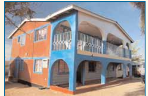
The new building at Timboni Tiva Children's Home
